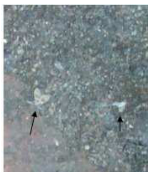
Figure 2 Sand flies on unplastered wall
